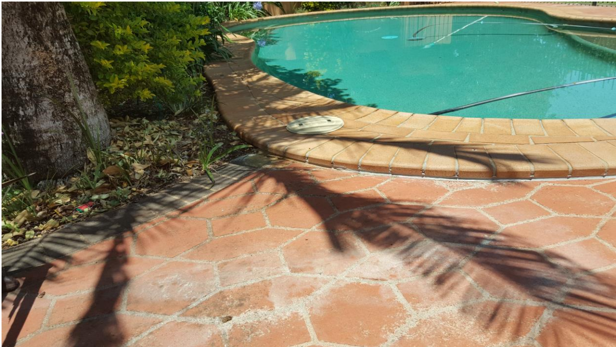
Pool coping to apron joint after -10mm
