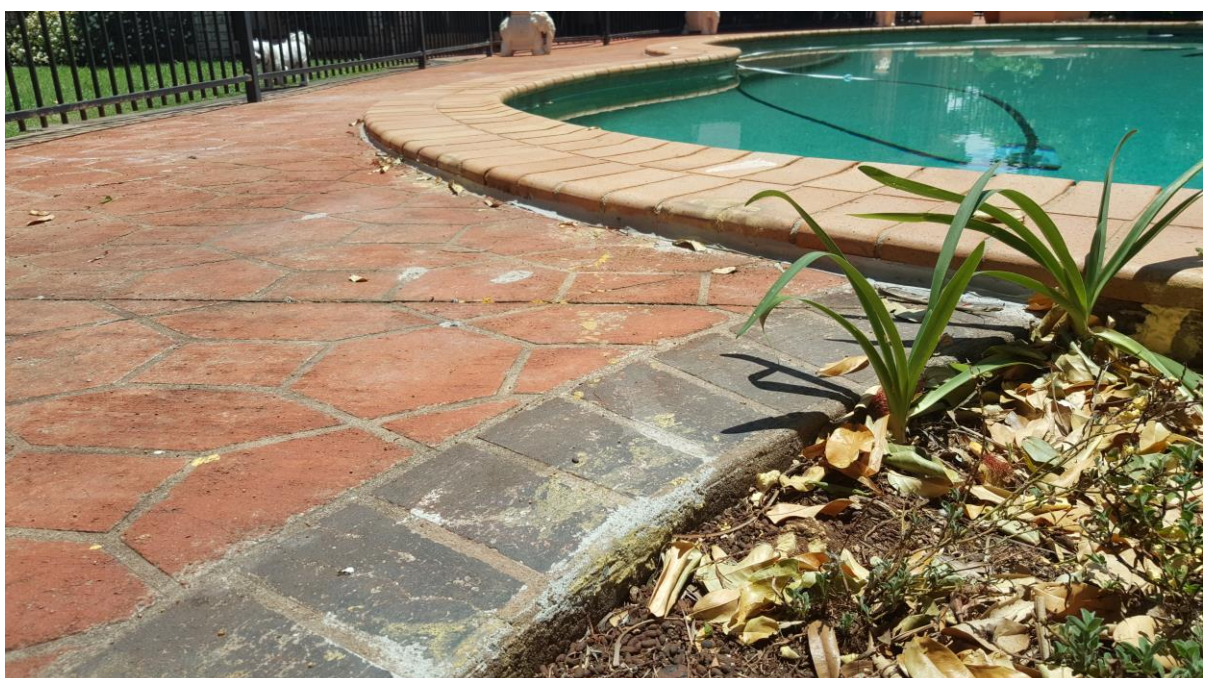
Pool coping joint after -10mm, was originally -70mm
